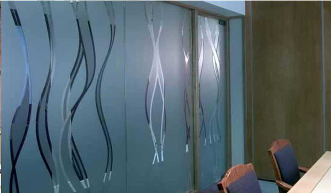
*Vision panels of almost any shape or size can be incorporated to conform with building regulations and fire officer requirements.*
